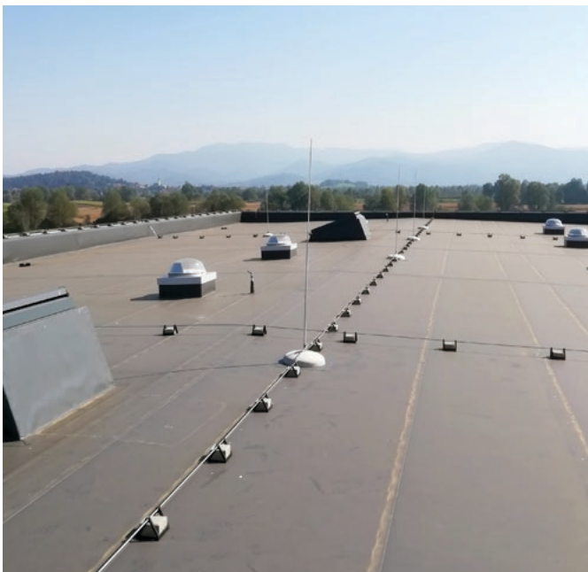
Figure 12: Catching rod mounted on a flat roof
