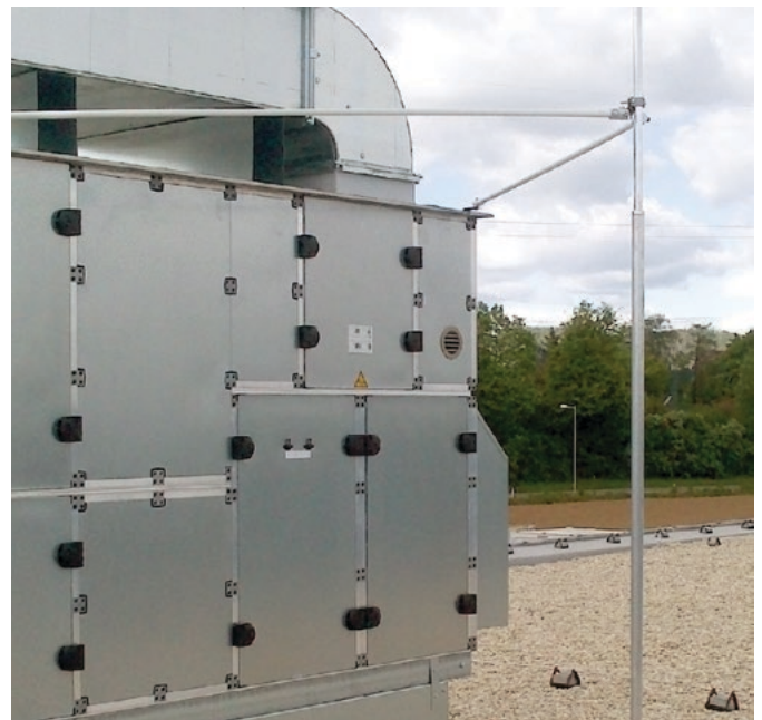
Figure 13: Catching rod mounted on a flat roof and additionally attached to the protected device by means of spacer elements.
