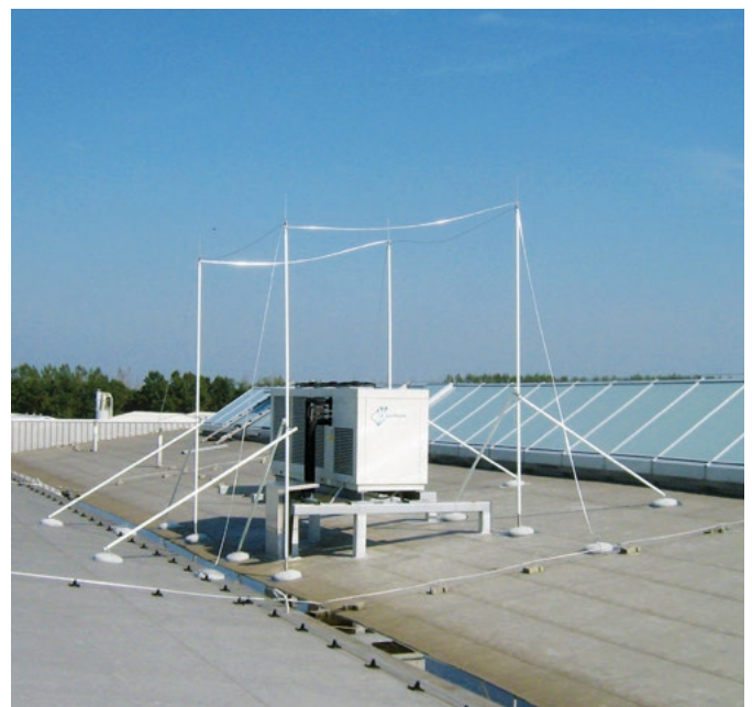
Figure 15: Catching system mounted on insulated load-bearing elements IZ045
