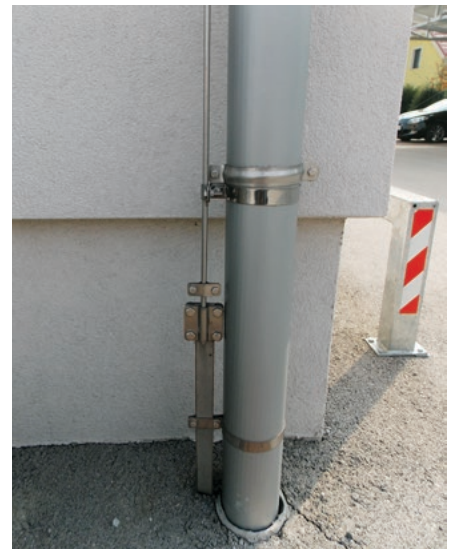
Figure 17: Downconductor, installed on the drain pipe
