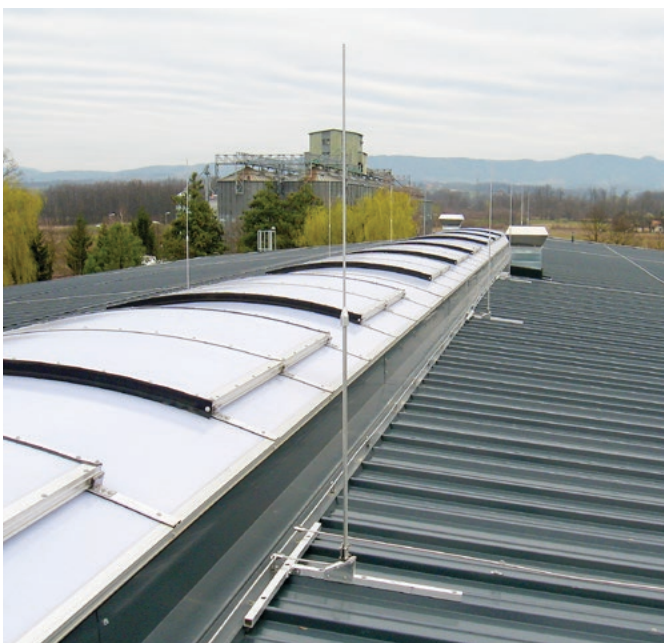
Figure 14: Catching rod mounted on the roof covered with trapezoidal tin sheet roofing
